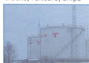
Tank Management Systems
